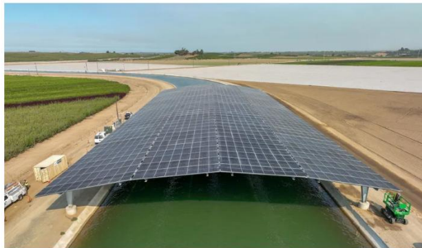
The roughly 110-foot-wide portion of the canal-top solar project near Hickman, California. (Turlock Irrigation District)
