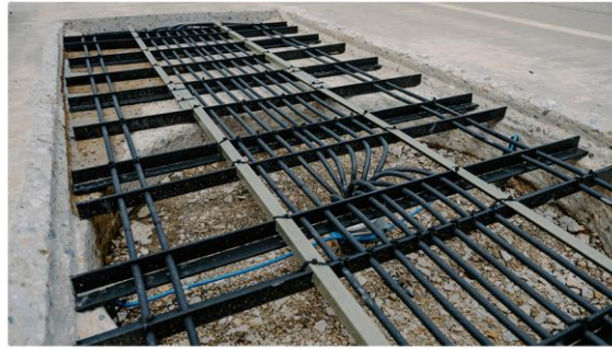
The Indiana Department of Transportation embedded these Purdue-designed coils before covering them with concrete highway pavement. The coils transmit power to receiver coils attached to the underside of an electric heavy-duty truck. (Purdue University photo/Kelsey Lefever)
